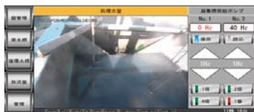
Remote control screen for volume of water treated
