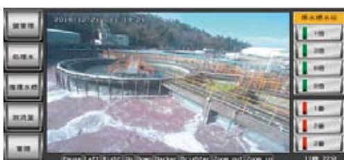
Wastewater treatment equipment area monitoring screen
